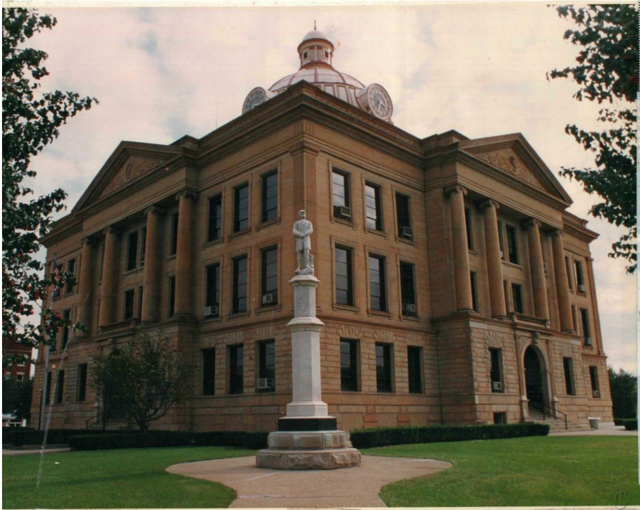
1905 Logan County, Illinois Court House before current restoration project, pre-2008.
